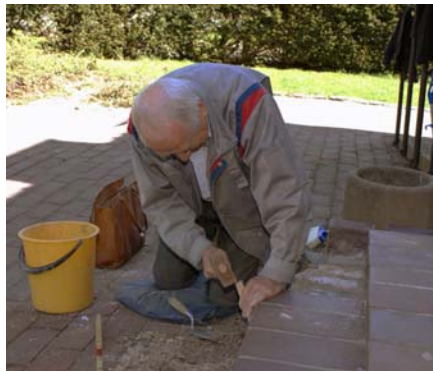
Bank Bank Bank Krash ...Hoppsan!
